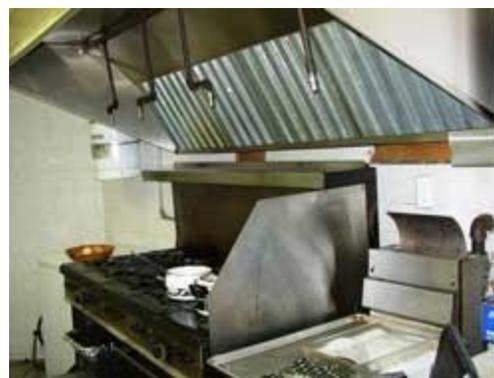
This photo illustrates the correct installation of a metal baffle plate between the open flames from the range and the deep fat fryer. Metal baffles should be used only when there is not sufficient space available to provide a 16-inch clearance between the deep fat fryer and any source of open flames.
