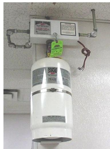
These photos are examples of two different brands of automatic extinguishing systems that contain a liquid extinguishing agent. Ansul and Range Guard are two well-known manufacturers. Also, note the inspection tag on the unit to the left. This is the inspection tag that the servicing company will leave after they service the system every six months.
