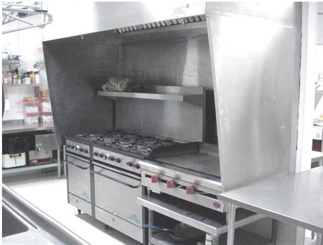
The photo to the left is an example of kitchen appliances that are properly equipped with an appropriate hood and ventilation system.
