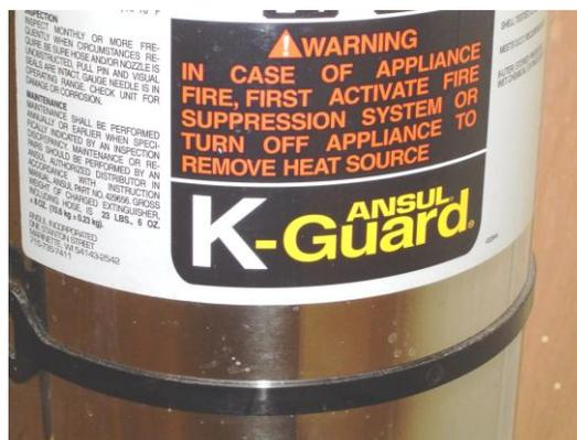
These pictures are of a portable K-rated fire extinguisher. A class K fire extinguisher is designed to better control grease and other kitchen related fires. If a kitchen contains any grease producing appliances, a portable Class K-rated fire extinguisher should be installed in the kitchen in a visible and easily accessible location.
