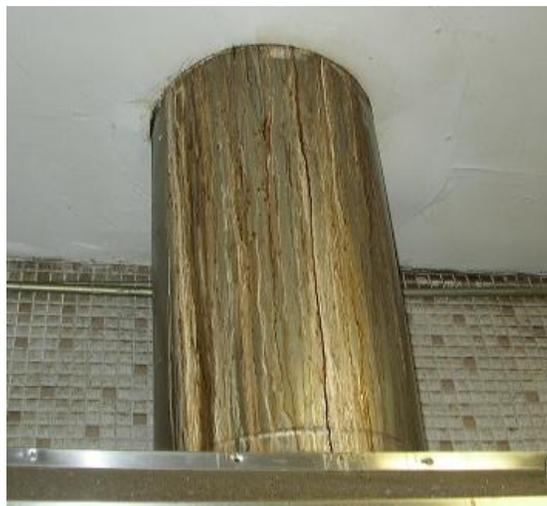
This photo shows ductwork from a cooking area that has a heavy accumulation of grease. Maintaining and cleaning the hood and ventilation system is crucial, as the buildup of grease can become a serious fire hazard. The hood and ventilation system should be inspected and cleaned by a certified contractor every six months.
