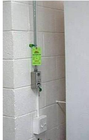
These photos are examples of manual activators that should be used if the automatic extinguishing system fails to activate. This device should be installed away from the cooking surface, next to an entrance/exit for the kitchen. Kitchen staff should be aware of this manual activator and trained on its use. Also note the inspection tag. Many fire service companies will place these tags on the manual activator to indicate current servicing.
